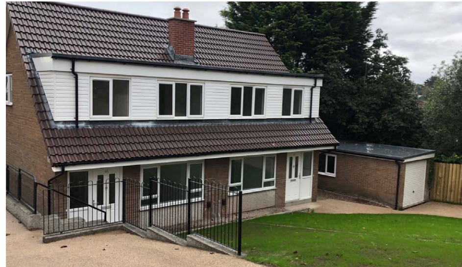
House in Mountview, Lisburn, which was renovated.
