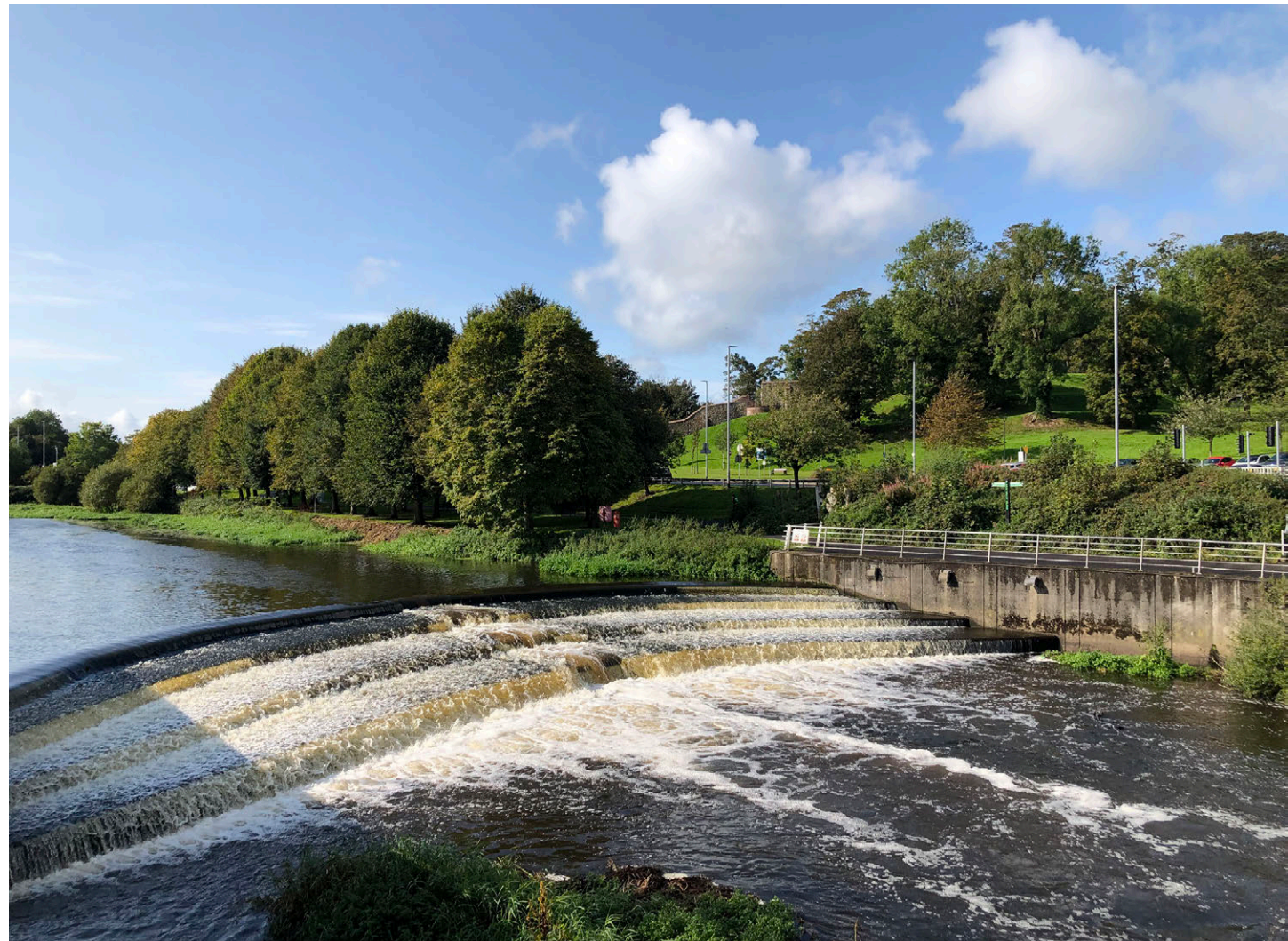
Weir, Lagan Valley Island, Lisburn
